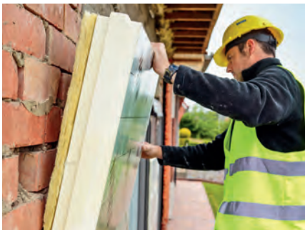
UTHERM Wall flex PIR L | λ 0,022 W/mK Velikost desek: 600 mm x 1200 mm
